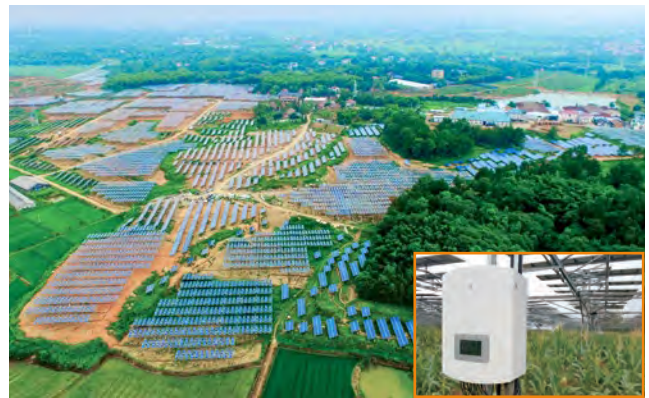
Zhejiang Quzhou Agricultural-photovoltaic hybrid PV plant 20MW
