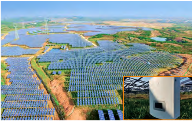
Zhejiang Hangbu Agricultural-photovoltaic hybrid PV plant 30MW
