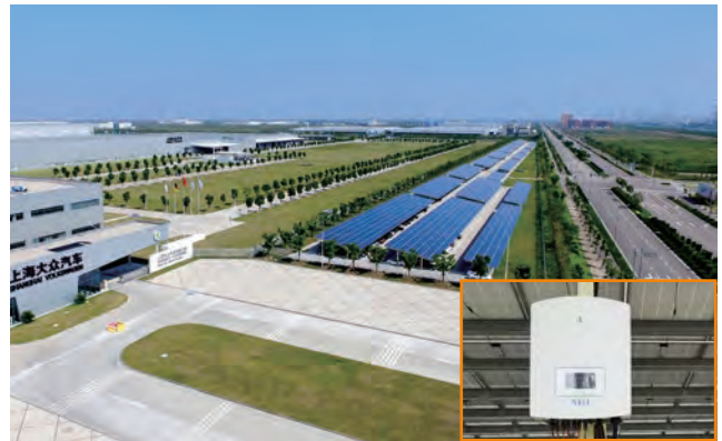
Shanghai Volkswagen Photovoltaic solar carport 55MW
