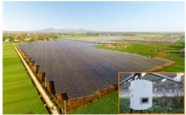
Hubei Guanyin Agricultural-photovoltaic hybrid PV plant 20MW
