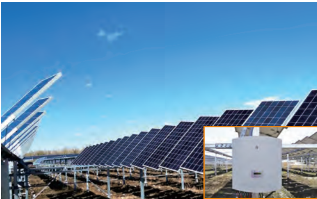
Hebei Zhangbei Agricultural-photovoltaic hybrid PV plant 50MW
